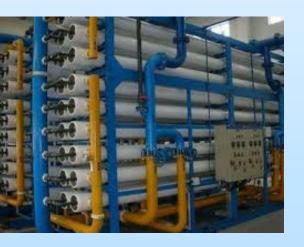
Bio fouling control at the inlet of RO membranes.
